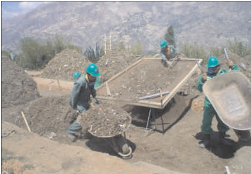
Organic waste treatment plant of the Provincial Municipality of Carhuaz: organic waste is transformed into compost and humus for agricultural purposes.
