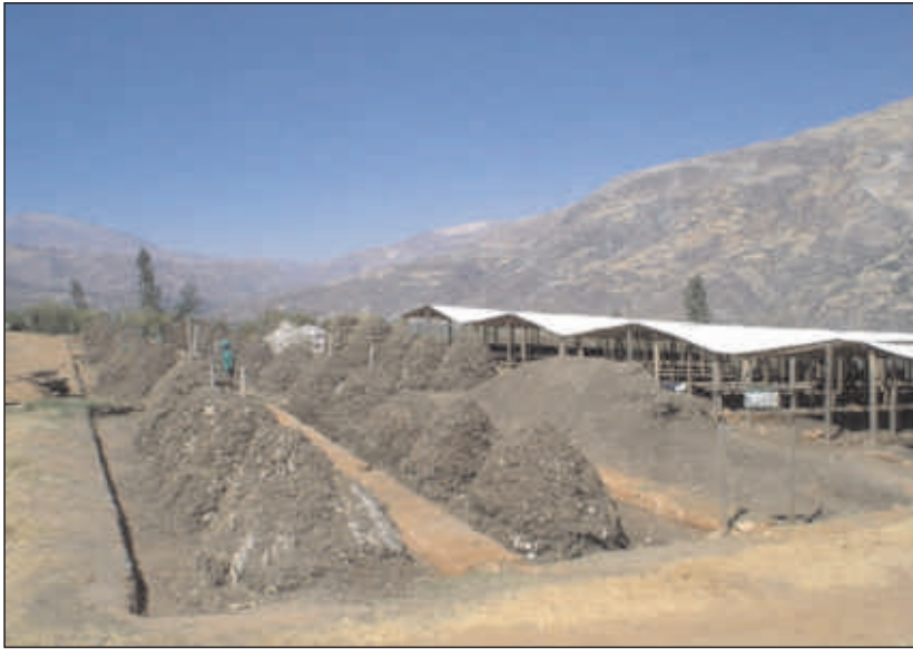
Organic waste treatment plant of the Provincial Municipality of Carhuaz: organic waste is transformed into compost and humus for agricultural purposes.
